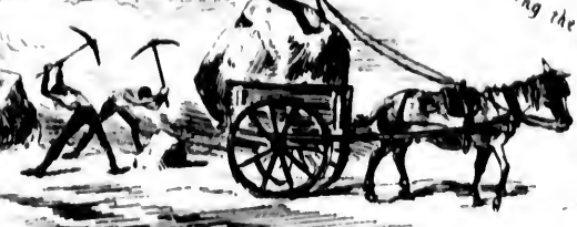
Clearing away rubbish &c.
