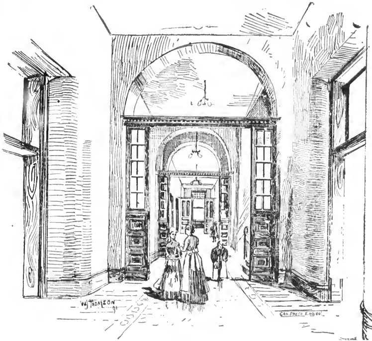
MAIN CORRIDOR—FIRST FLOOR.
