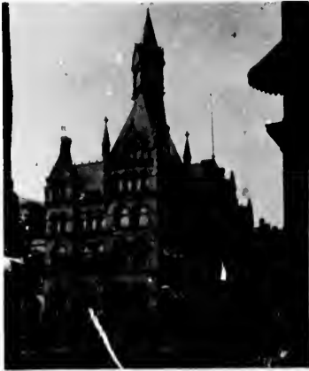
The Canada Life Building, at Hamilton.
