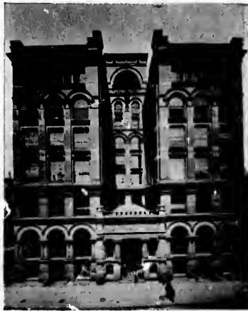
The Canada Life Building, at Toronto.
