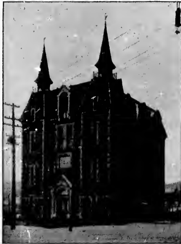
WESTERN HOSPITAL, MONTREAL.
