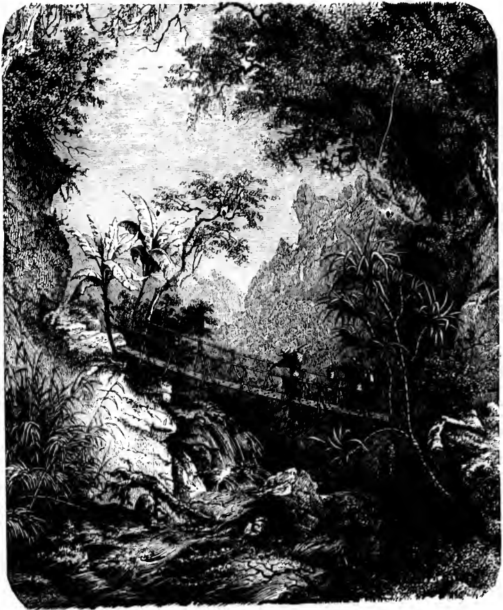
BRIDGE NEAR KABADI.
