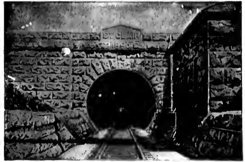
The St. Clair Tunnel.
