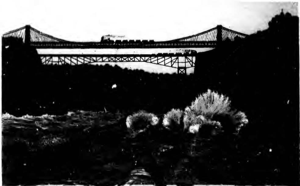
WHIRLPOOL RAPIDS - RAILWAY SUSPENSION BRIDGE AND CANTILEVER BRIDGE
