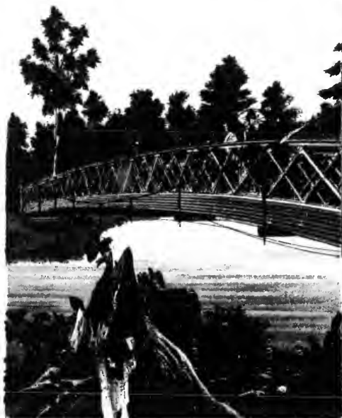
BRIDGE TO SECOND SISTER ISLAND.
