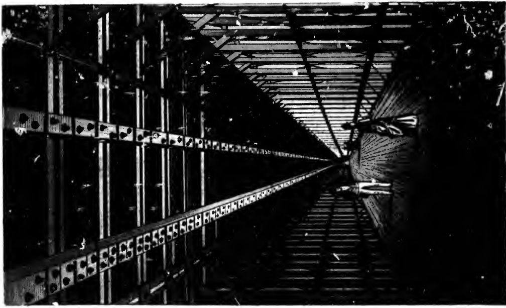
INTERIOR RAILWAY SUSPENSION BRIDGE 800 FEET LONG
