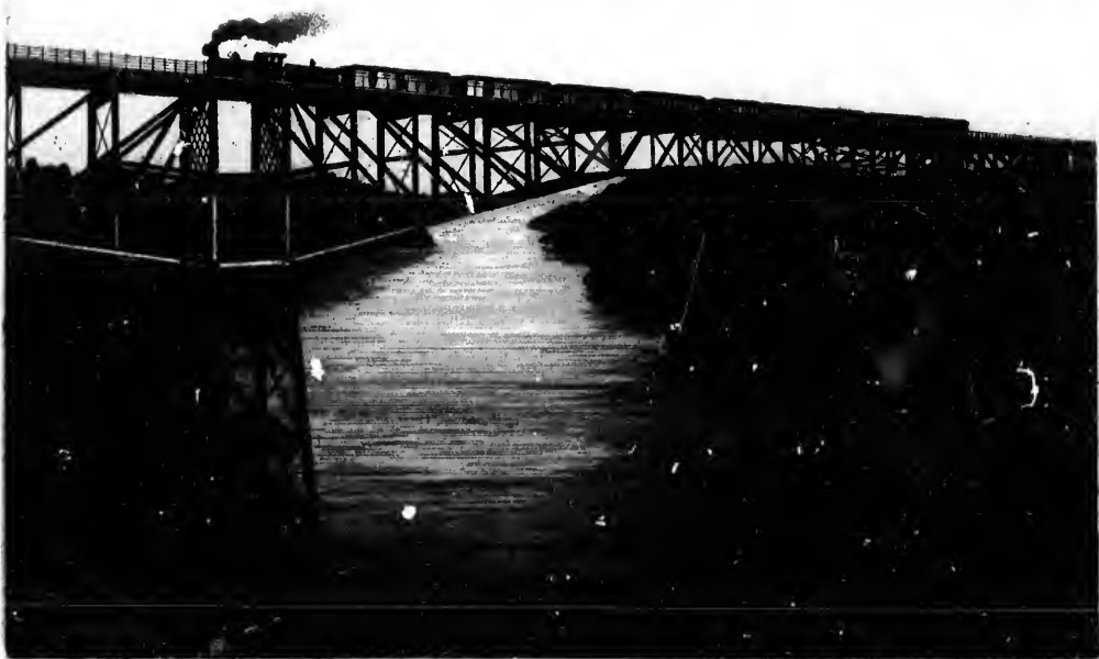
CANTILEVER BRIDGE MICHIGAN CENTRAL R.R.
