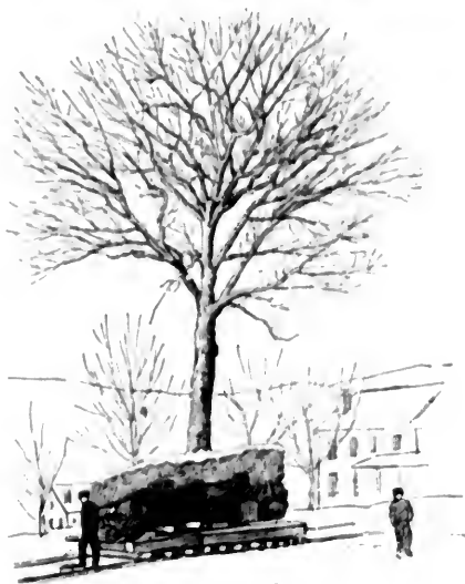
2546. Moving a tree in winter, with a large ball of frozen earth.
