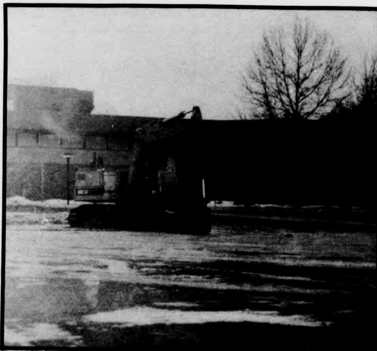
The site of the York Lanes development
