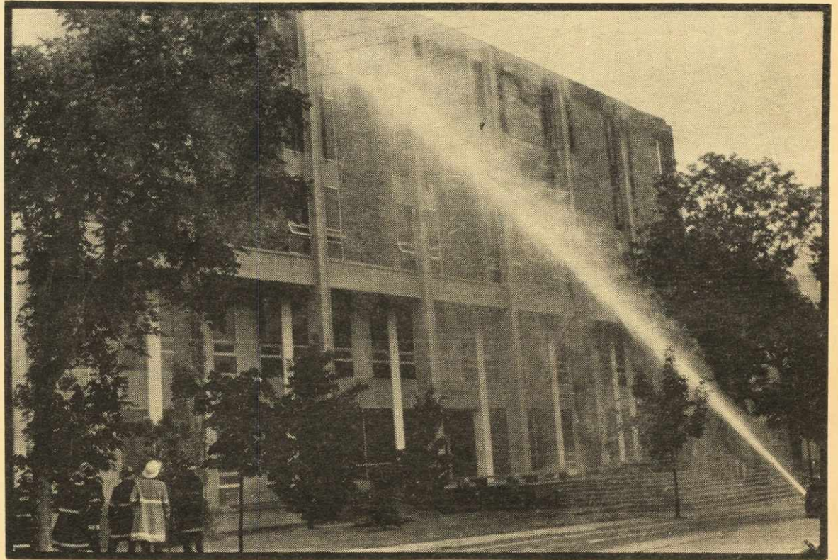
Firefighters battle Weldon blaze, result of lightning strike. The fire destroyed the fifth floor and caused heavy damage to the fourth. Dal Photo: Valerie Berryman
