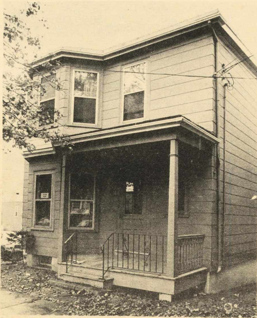
Students of Dalhousie's lower campus find fleeting happiness in Carleton House. The house, newly renovated, is soon to be taken away.
