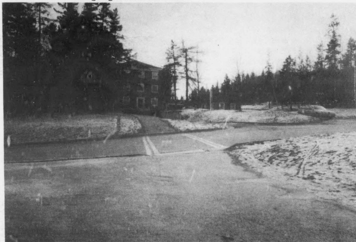
These photos demonstrate the problem of inaccessibility at one of UNB's many trouble spots. The photo above shows the sloping of some of UNB's paths and walkways which makes them prone to cracks, potholes and ice patches (note particularly the dip in the walkway leading towards Kierstead Hall, immediately in front of the Harriet Irving Library). The photo below shows the curb and upward-sloping sidewalk which wheelchair users would run into going towards the SUB.
