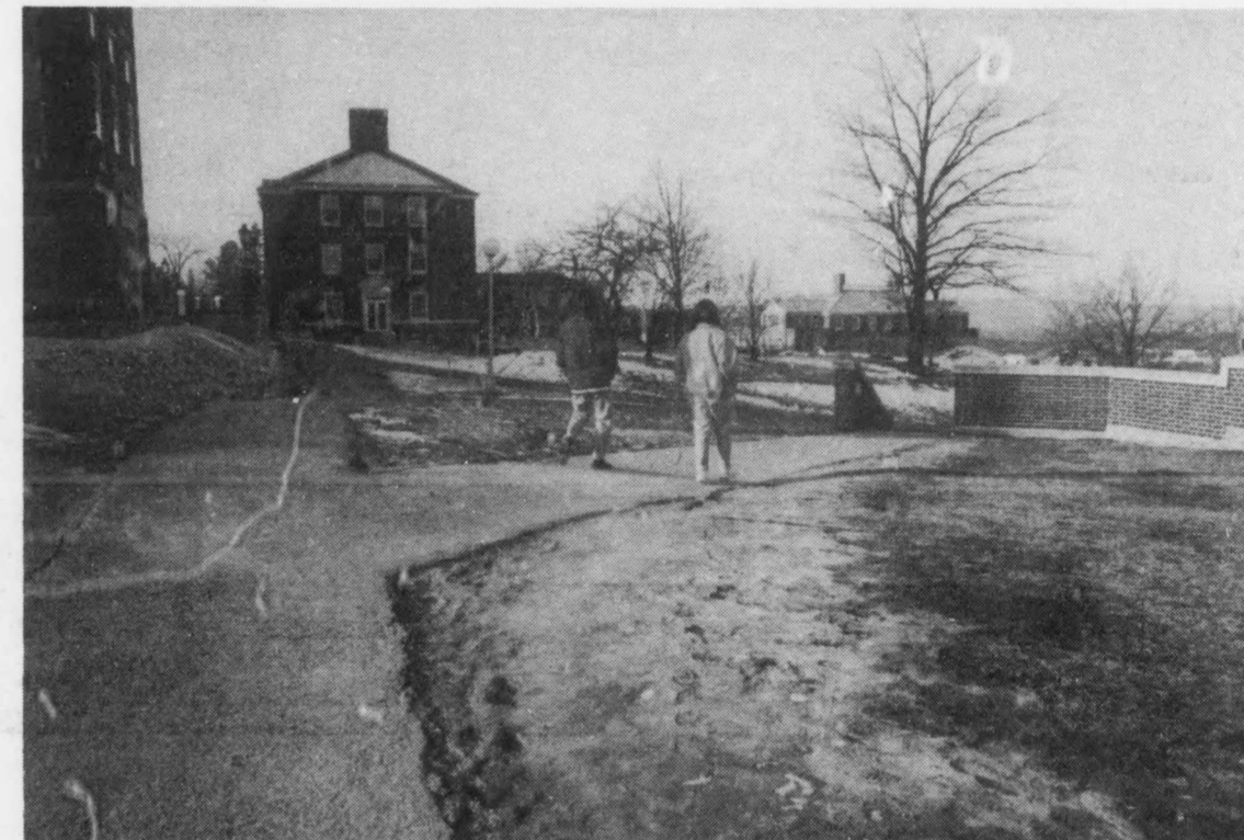
These photos demonstrate the problem of inaccessibility at one of UNB's many trouble spots. The photo above shows the sloping of some of UNB's paths and walkways which makes them prone to cracks, potholes and ice patches (note particularly the dip in the walkway leading towards Kierstead Hall, immediately in front of the Harriet Irving Library). The photo below shows the curb and upward-sloping sidewalk which wheelchair users would run into going towards the SUB.
