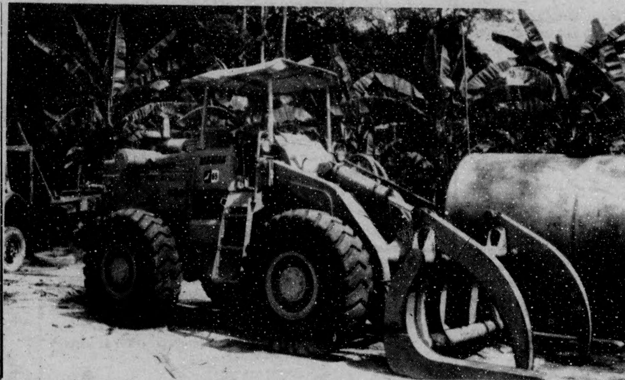
Loaders replacing the pulley system
