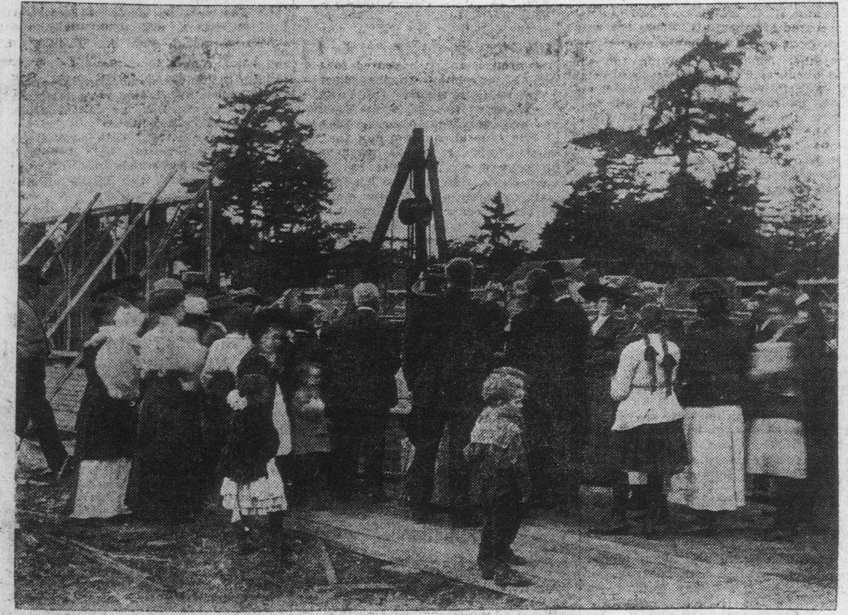
LAYING CORNER STONE OF NEW SCHOOL ON MOSS STREET ON MONDAY AFTERNOON
