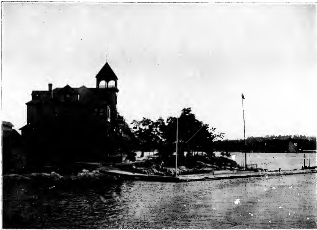
PULLMAN HOUSE, GERNELL PARK.
