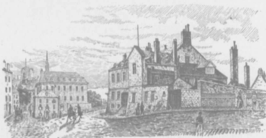
Chateau Haldimand, Quebec, 1784. Demolished in 1892 to give place to the Chateau Frontenac Hotel
