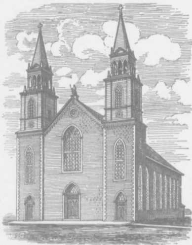
Church of Saint-Roch des Aulnaies.
