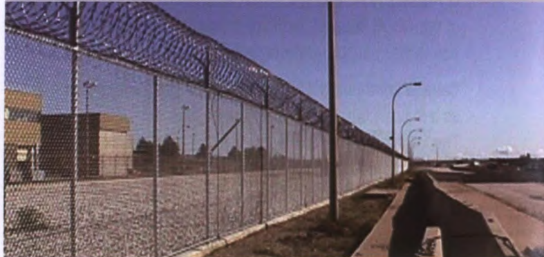
Perimeter security fences help ensure that terrorists do not gain access to dangerous nuclear materials. Photo Credit: Canadian Nuclear Safety Commission
