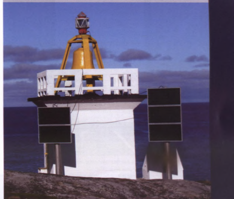
Solar cell panels provide a sustainable alternative power source for lighthouses formerly powered by highly radioactive material. Photo Credit: County Governor of Finnmark (Norway)
