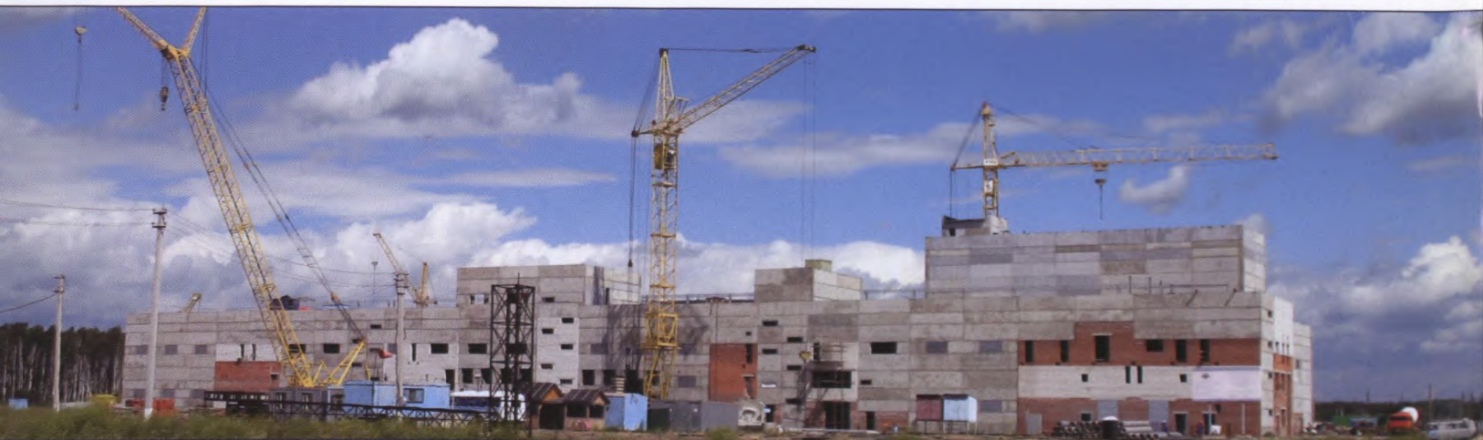
Second main destruction building, Shchuch'ye chemical weapons destruction facility
