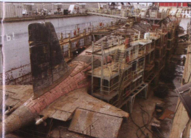
Victor I being dismantled in floating dock
