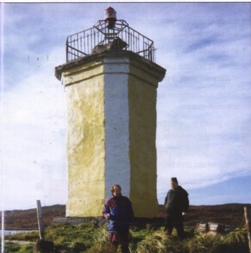
Lighthouse powered by radioisotope thermoelectric generator (RTG) containing highly radioactive material. Photo Credit: County Governor of Finnmark (Norway)
