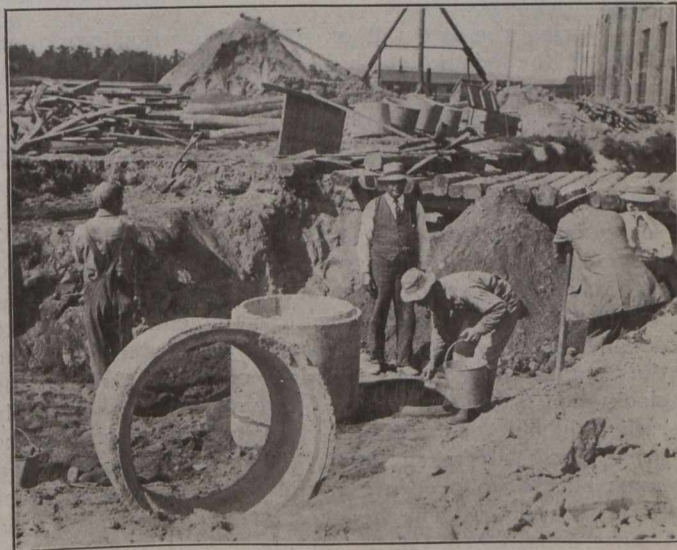
Fig. 8—Constructing Manholes with 30" Concrete Pipe.
