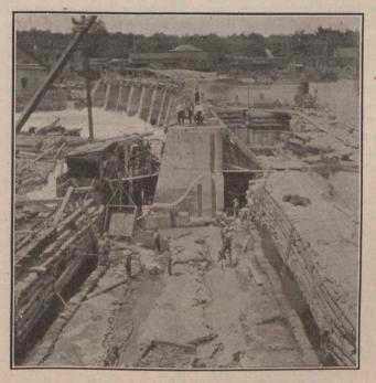
Fig. 3.—Showing Cofferdam After Pumping.
