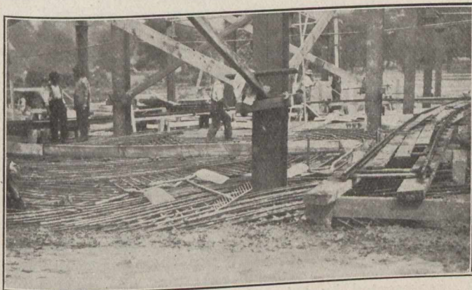
Reinforcement in place.
