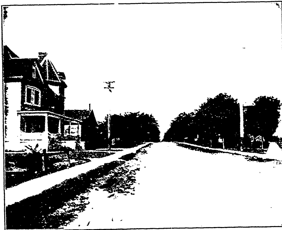
Residential Street Albert Street
