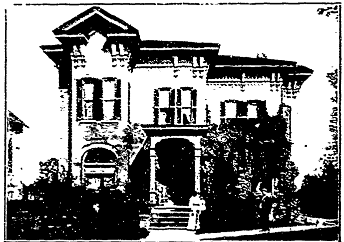
Residence of Dr. A. F. Bauman, King St.
