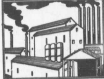
Our mills are located all over Canada, so that no matter where you live you can get Canada Cement without paying high prices caused by long freight hauls.
