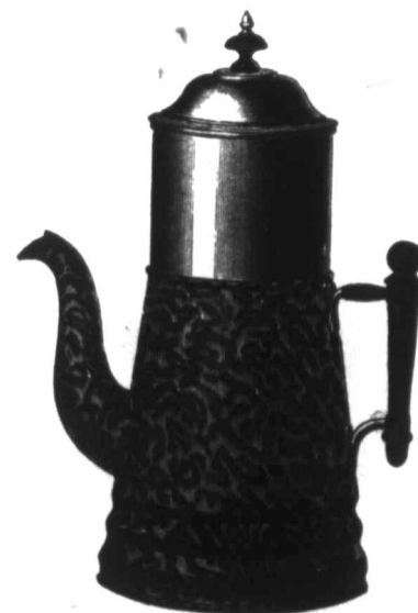
French Coffee Biggin—With Polished Tin Filters and Asbestos Cushion Copper Bottoms
