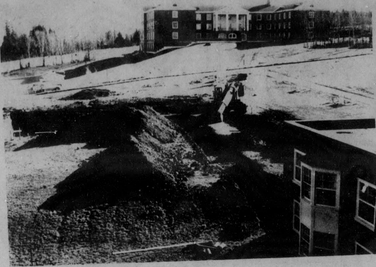
Construction has begun on MacKenzie house the new men's residence that will house 100 men in 30 single and 35 double rooms. The residence will complete the Jones, Neil, and Bridges Quadrangle.
