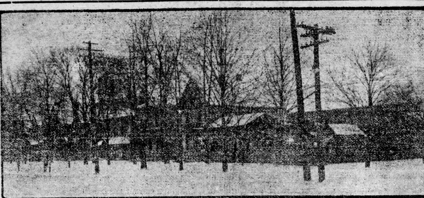
Photo by The Advertiser Photographer. The cut is made from a picture looking west from the corner of King and Waterloo streets. All the buildings in the picture will be bought and torn down.
