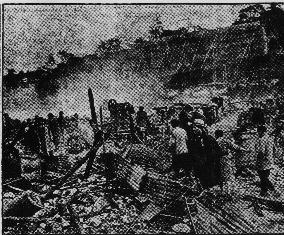
Fire, starting from sparks of a charcoal fire in a pan, with which Japanese wood and paper dwellings are heated, consumes 250 houses at Kita Shinjima, Tokyo suburb. Photo shows native Japanese looking for their belongings.
