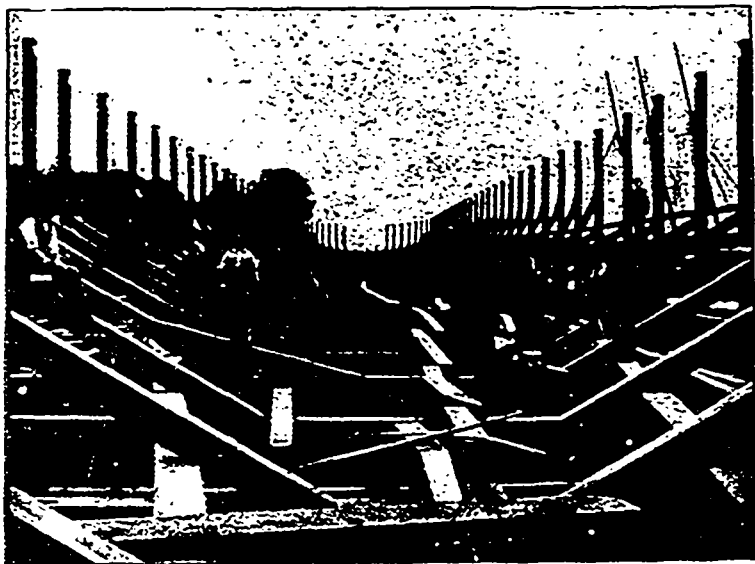
A CRADLE IN PROCESS OF CONSTRUCTION, BEFORE LAUNCHING.
