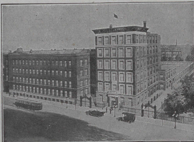
FIRE PROOF BUILDINGS
