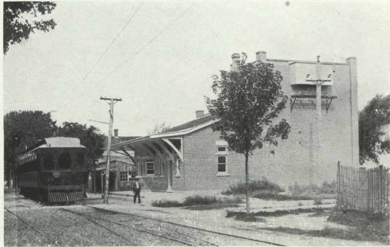
THE RADIAL STATION
