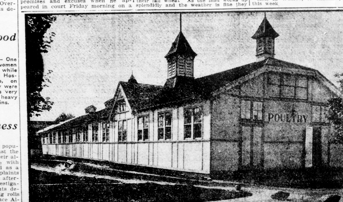
ENLARGED POULTRY BUILDING A THE WESTERN FAIR.
