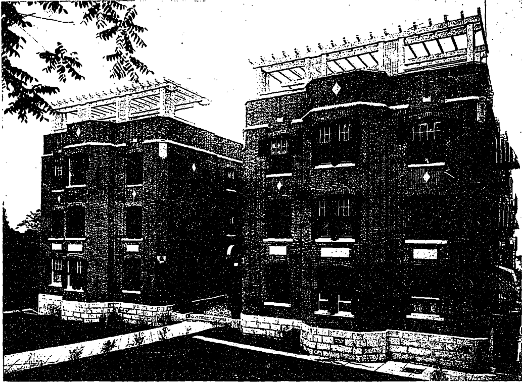
An Unusual Adjunct of the "Travancore" is a Roof Pergola an Excellent View of which is Obtained Herewith. This Innovation Suggests Certain Possibilities in "Roof Gardening" which Might Well be Considered by Architects in Providing Outdoor Advantages, Especially where the Ground Dimensions are Restricted on All Sides.
