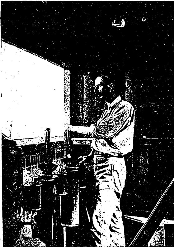
One of the Cableway Operators in His Booth, Showing the Simple Apparatus with which He Controls the Operation of the Bucket and Carriage.
