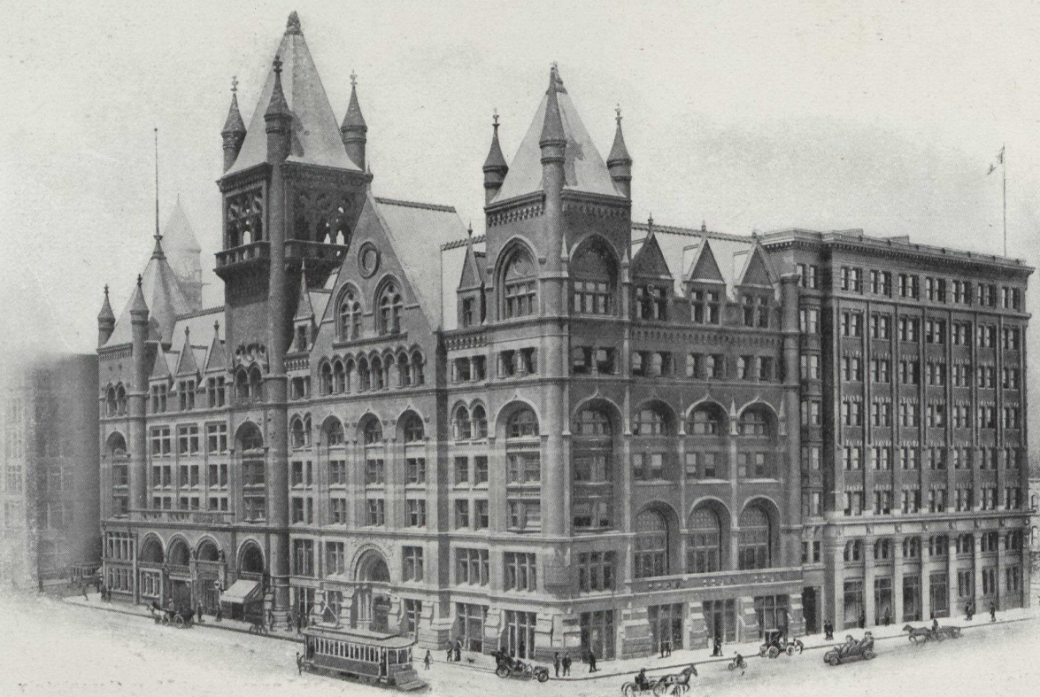
THE CONFEDERATION LIFE BUILDING, TORONTO, SHOWING THE NEW ADDITION RECENTLY COMPLETED. WILSON J. GRAY, ARCHITECT. KEITH & FITZSIMONS, PLUMBERS. THIS NEW ADDITION TO ONE OF CANADA'S LARGEST OFFICE BUILDINGS IS EQUIPPED THROUGHOUT WITH PLUMBING WARE MANUFACTURED BY THE STANDARD IDEAL COMPANY, PORT HOPE, CANADA. NOTE.—IT WAS ERRONEOUSLY STATED, MUCH TO OUR REGRET, THAT THIS STRUCTURE WAS DESIGNED BY ANOTHER FIRM OF TORONTO ARCHITECTS.
