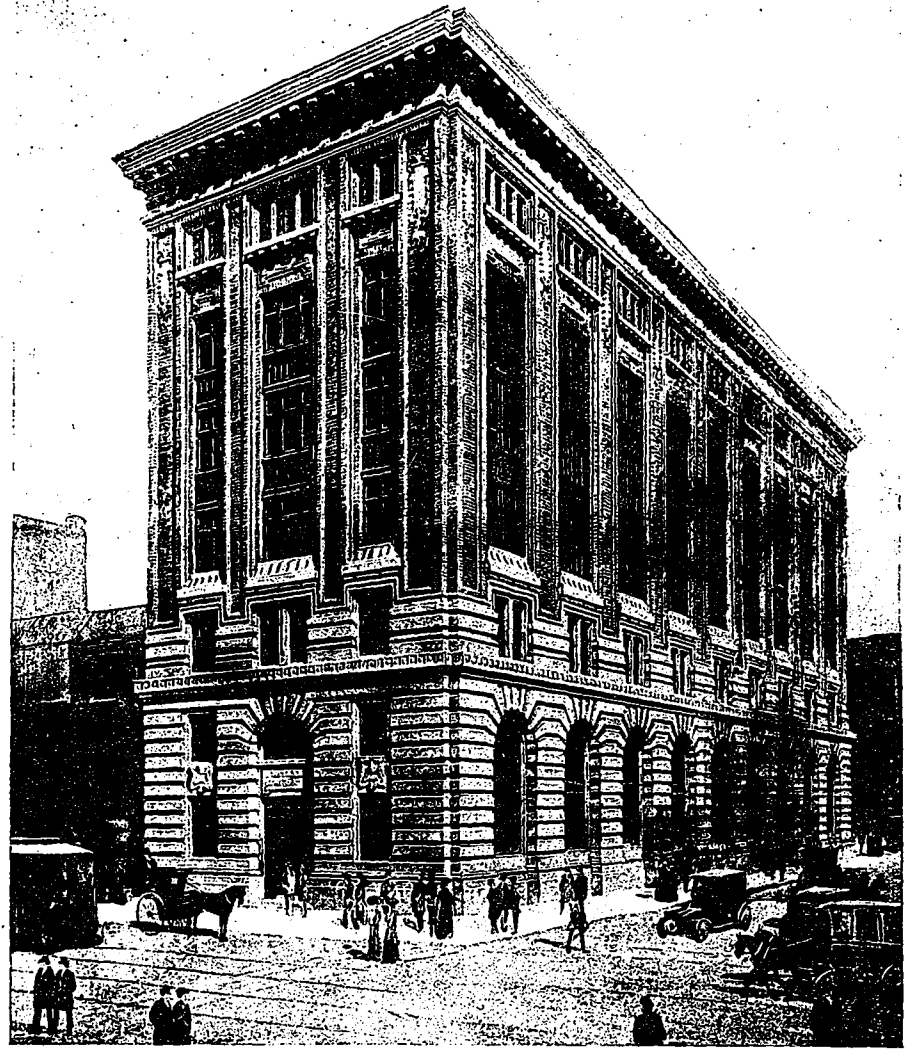
Design for Standard Bank Building, King St., Toronto, by Messrs. Darling and Pearson, Toronto.
