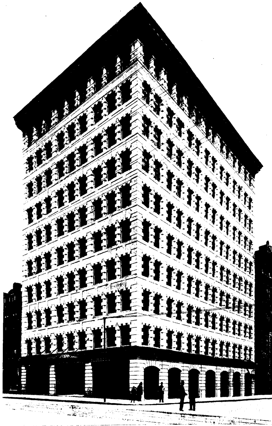
LUMSDEN BUILDING, TORONTO
