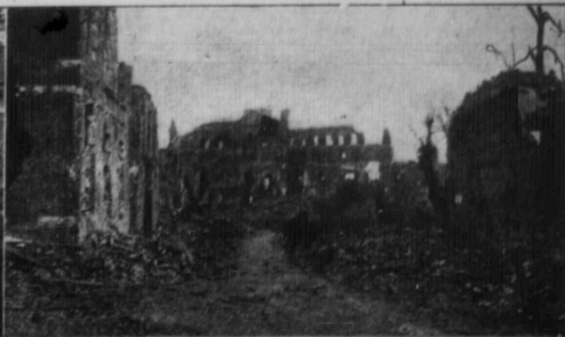
A View of the Ruins of the Church at Albert. A Characteristic Scene in the 'Fight-over Territory.'
