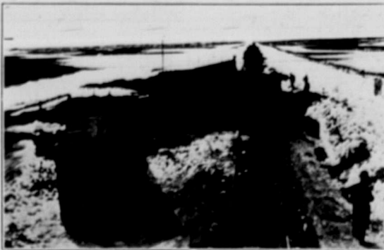
Result of broken rail on C.P.R. at Rindon siding, near Emerson, Man.
