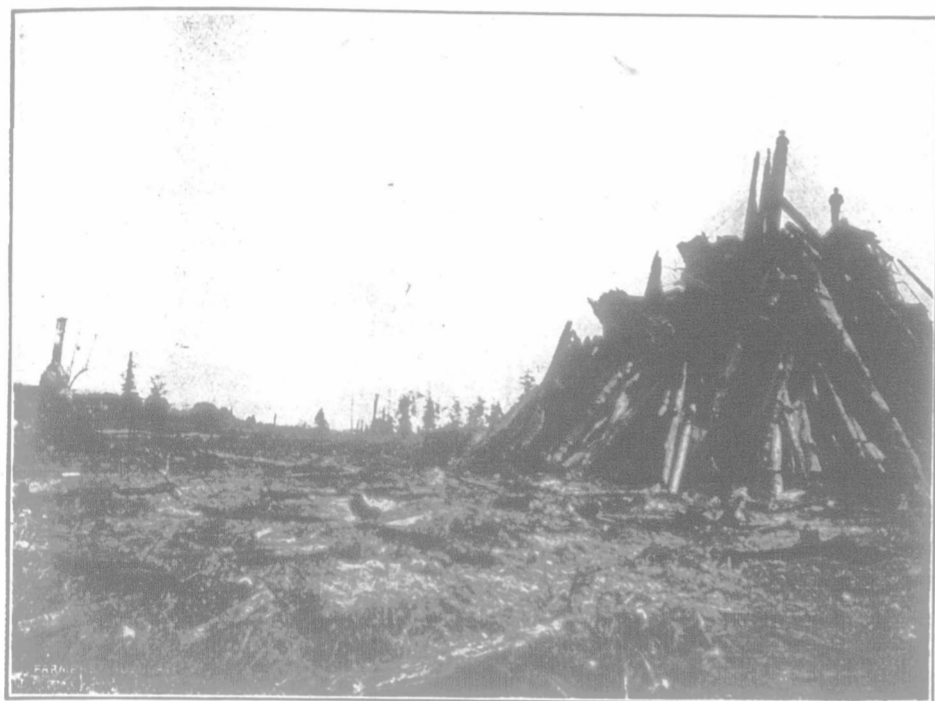
CLEARING LAND BY STEAM POWER
