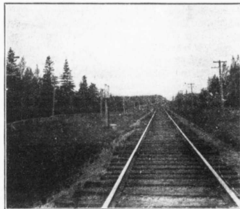
Fig. 1—Showing a Section of the I.C.R. Equipped with this System.
