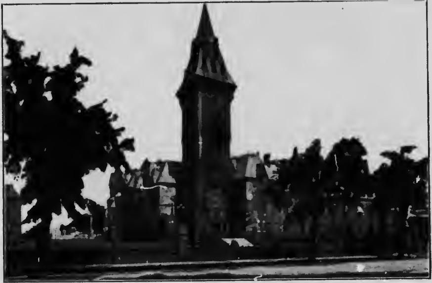
DEPARTMENTAL BUILDINGS—EAST BLOCK
