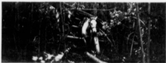
A Bad Stretch of Timber
