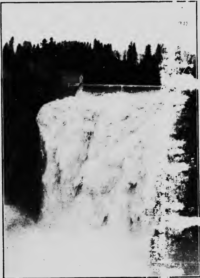
Montmorency Falls.—There are many good opportunities for the development of water powers in the St. Maurice River Valley, the St. Francis River Valley, the Lake St. John District, and the Abitibi District. See page 15.
