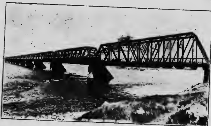
NEW VICTORIA BRIDGE.
