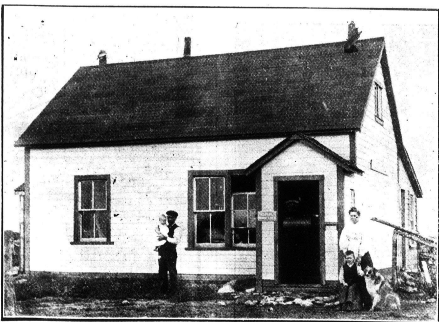
Pioneer Store, Post Office and C. P. R. Land Office just built at Manson, Man.
