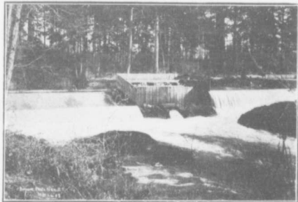
Nanaimo Electric Co's Dam.
