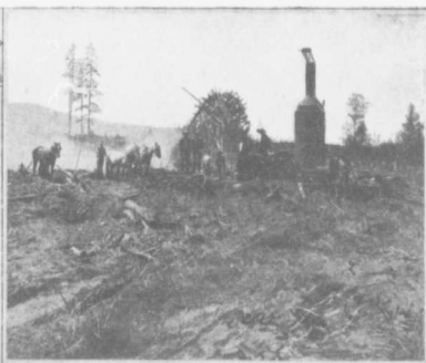
BAXTER'S LAND-CLEARING PLANT IN OPERATION
