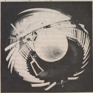
Technician installs closed-circuit television camera in isolation globe.
