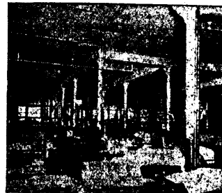
After Luxfer Prisms Installed.
