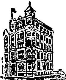
HEAD OFFICE BUILDING, MONTREAL.
