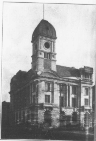
New Post Office, Regina, Saskatchewan, in course of construction.
