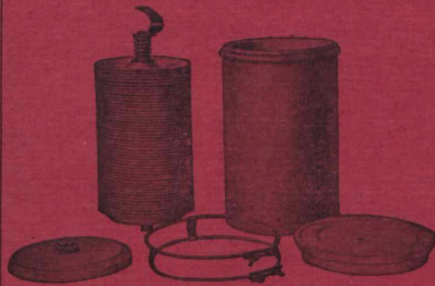
Type A Electrolytic Arrester, dismantled.
