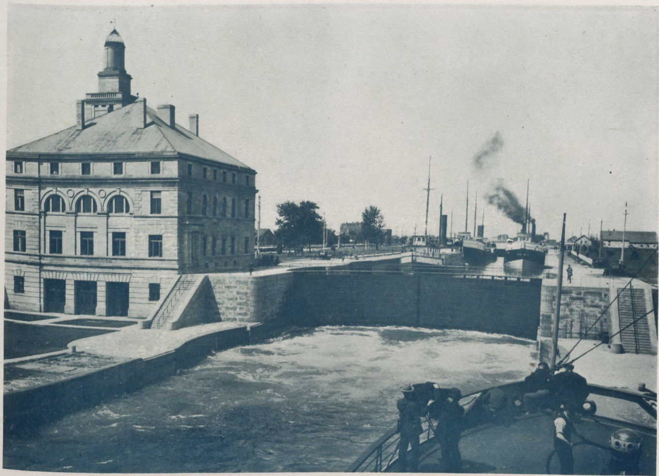
POE LOCK AND POWER HOUSE, SOO, MICH.
