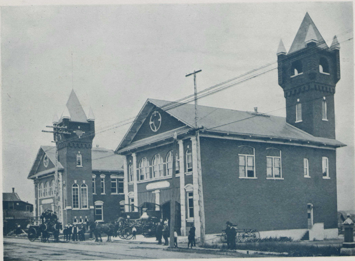
CITY HALL, CARNEGIE LIBRARY, MUNICIPAL BUILDING, FIRE HALL.
