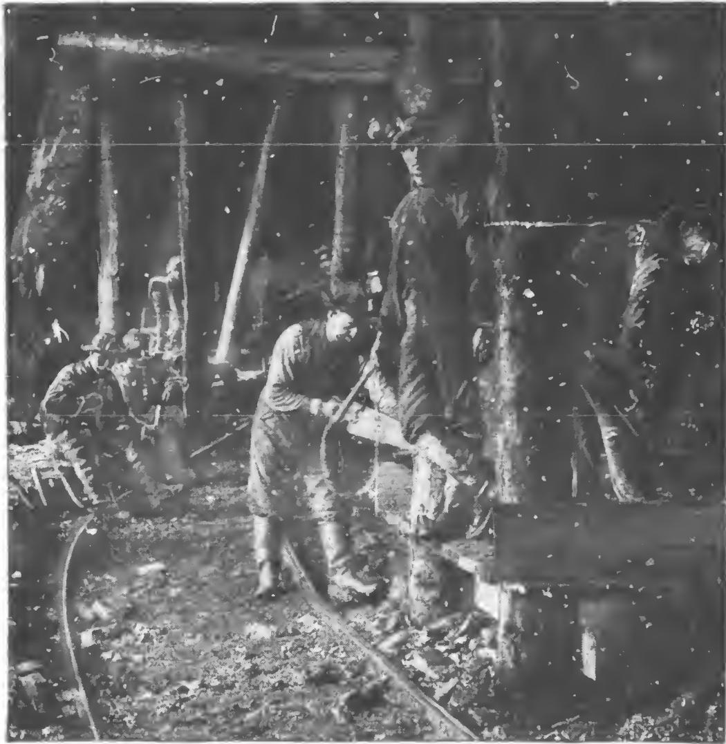
TIMBERMEN IN A GANGWAY.
