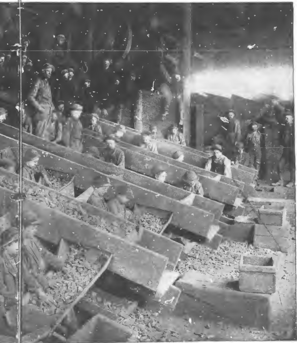
ROOM IN A BREAKER.
