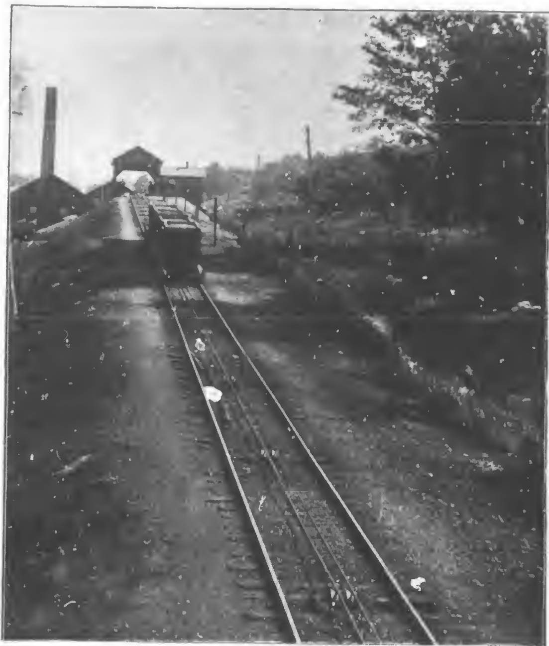
Plane on Gravity Road, near Carbondale.
