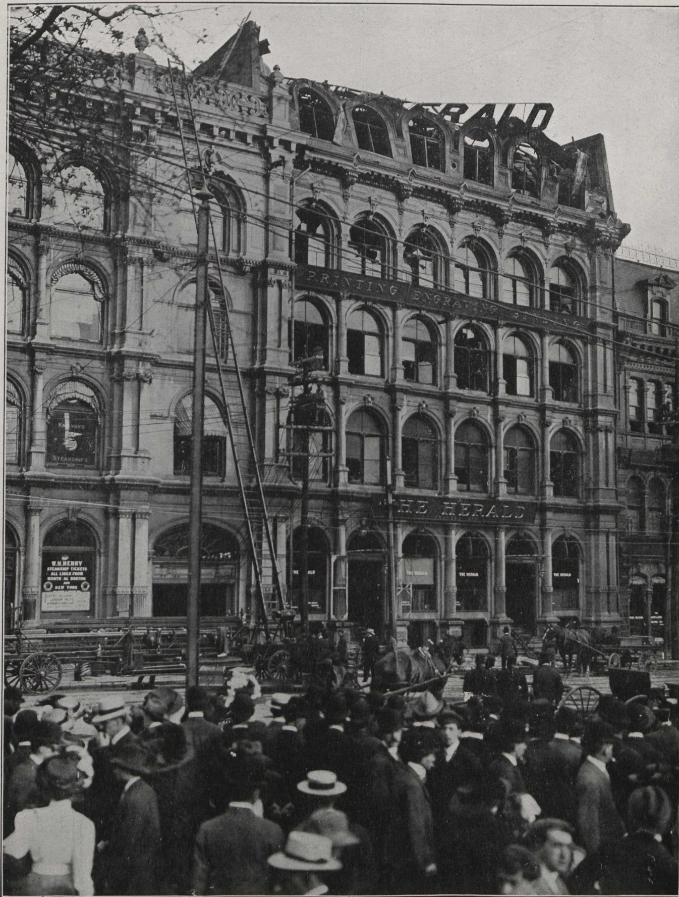
A Disaster that Cost Thirty-four Lives At half-past ten on the morning of Monday, June 13th, the water tank on the roof of the offices of the Montreal "Herald" collapsed and crashed through the five floors, burying itself in the basement with tons of debris, and, worst of all, nearly a hundred men, women, and girls. Some escaped almost unhurt, twenty-five were conveyed to the hospitals, and thirty-four bodies were taken out of the ruins. A score of these were heads of families. After the tank fell, with its sixteen thousand gallons of water, fire broke out, rendering the position of those still on the upper flats of the building one of the greatest danger. An investigation is being held to determine the cause, and place the responsibility.
