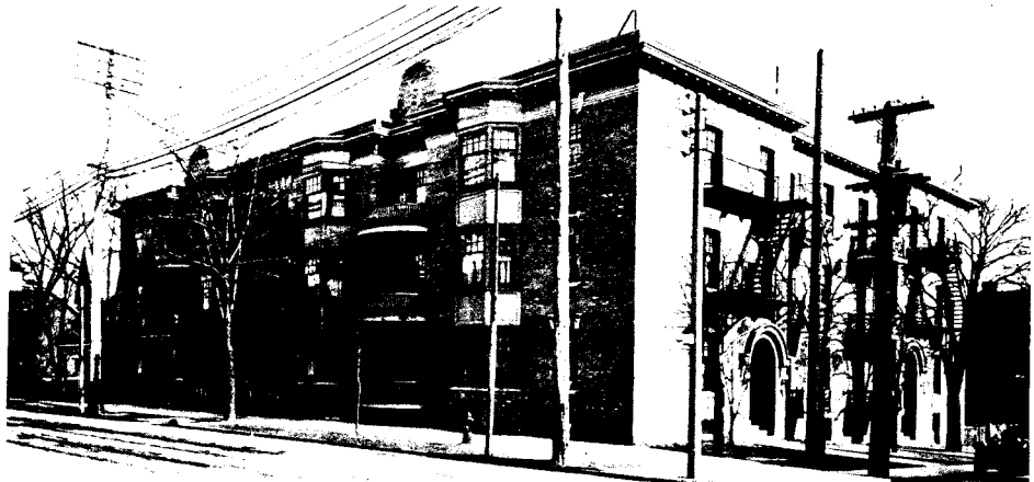
Park Apartments, Winchester and Metcalf Sts. Henry Simpson, Architect. Jas. Wickett, Ltd., Mason Contractors.
