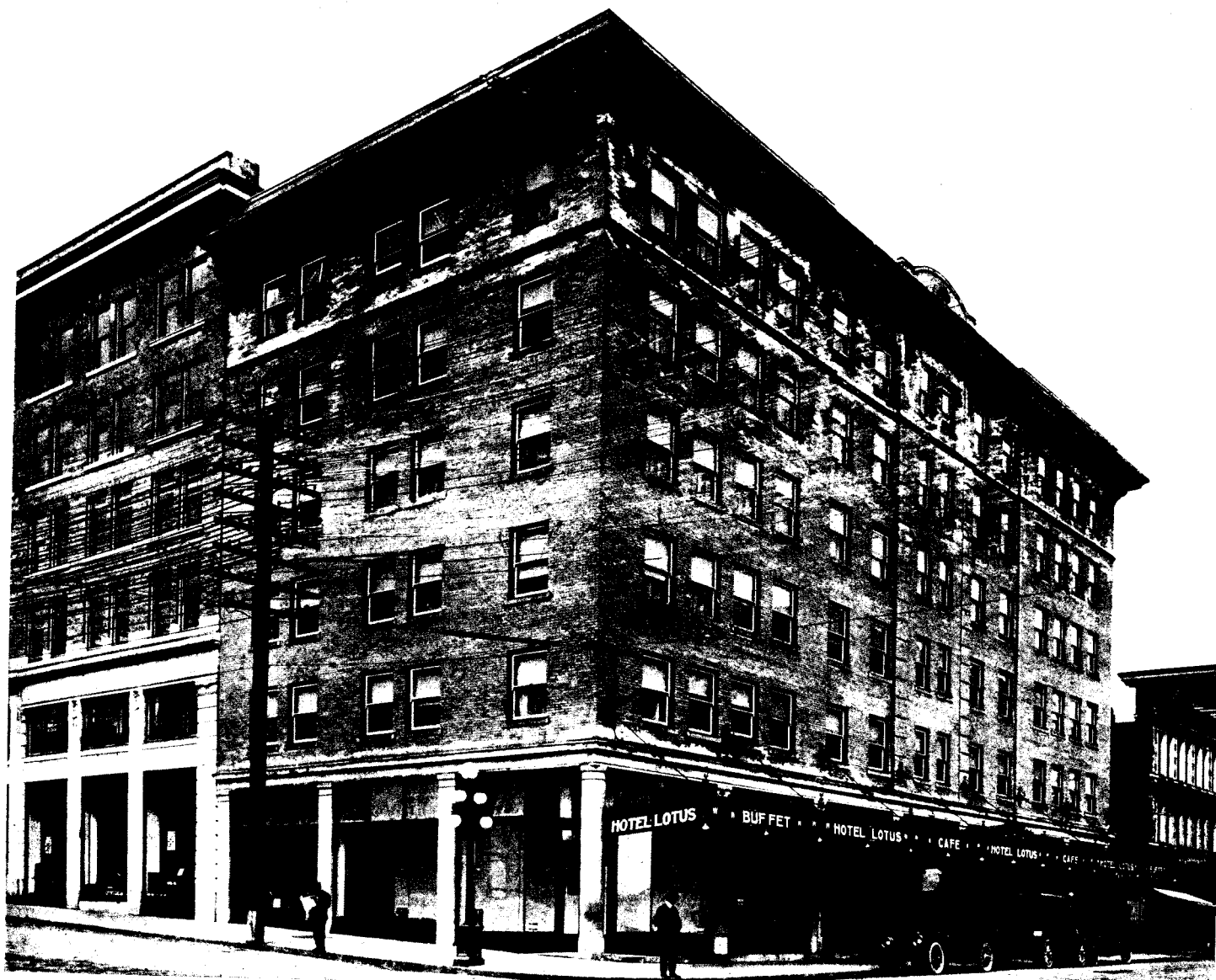
Hotel Lotus, Vancouver, B.C. Architect, A. J. Bird. Plumbers, Murray Bros. Contractor, R. McLean & Co. Standard Ideal Plumbing Fixtures used throughout.
