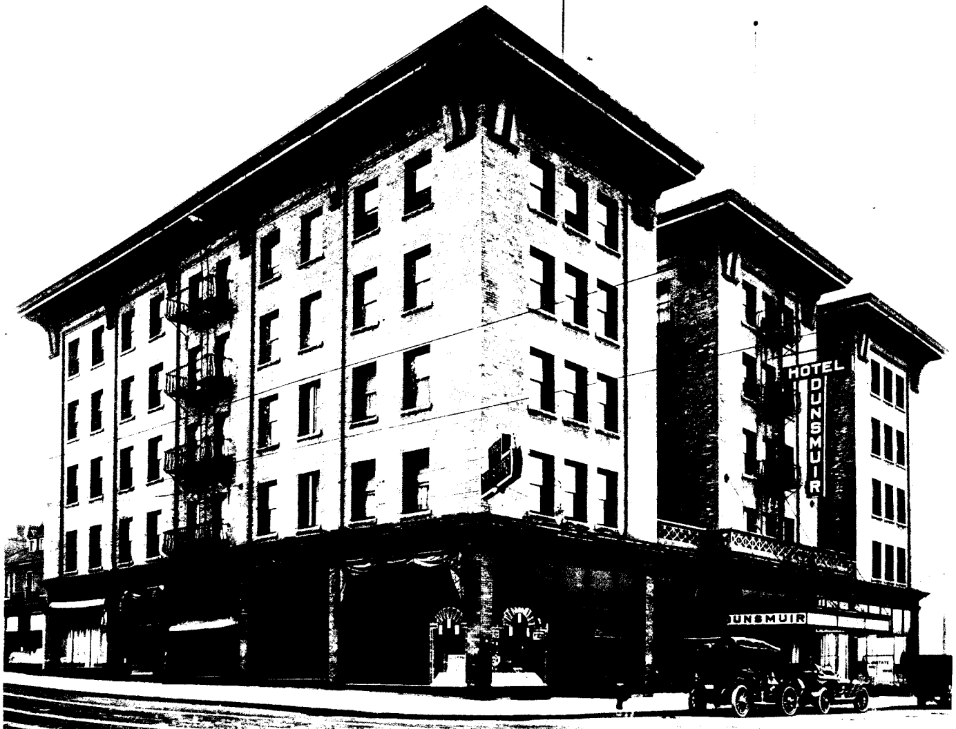
Dunsmuir Hotel, Vancouver, B.C. Architects, Parr & Fee. Plumbers, Barr & Anderson. G. W. Gibb, Contractor and Owner. Equipped with Standard Ideal Plumbing Fixtures.
