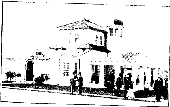
Residence of Mr. J. S. Stehlin, Long Beach, L.I. Covered with J-M Asbestos Stucco. Kirby, Pottit & Green, Architects.
