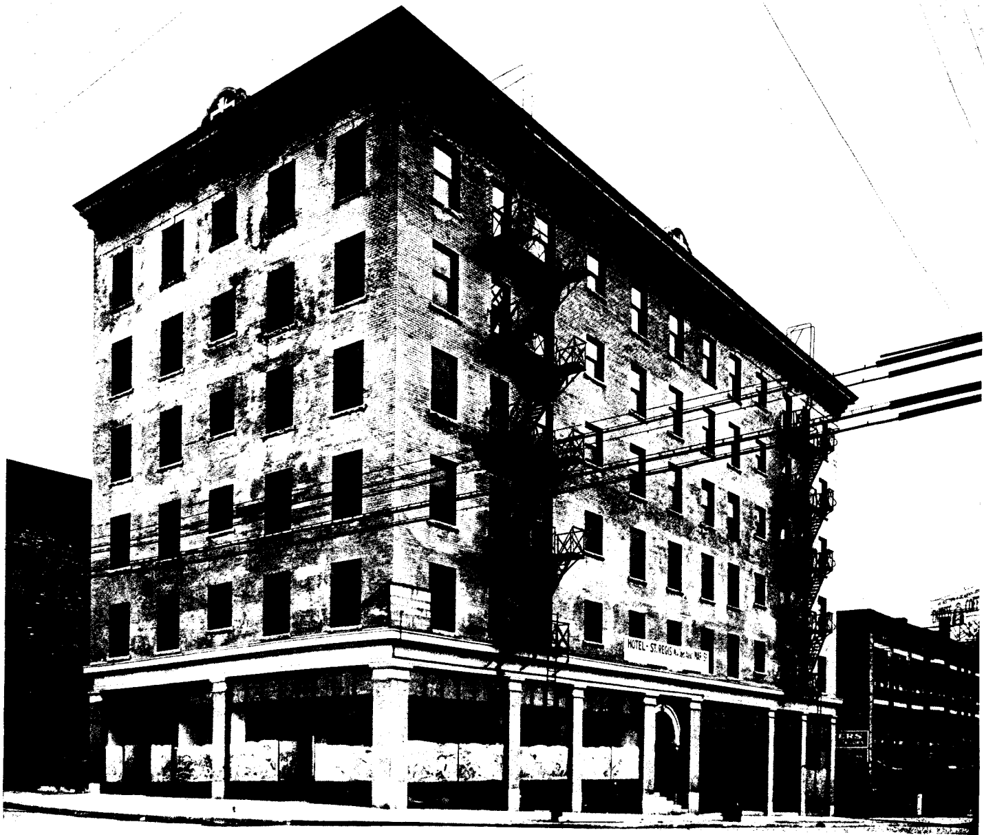
St. Regis Hotel, Vancouver, B.C. Architects, Dalton & Eveleigh. Plumbers, Barr & Anderson. Contractors, Baynes & Horie. Equipped with Standard Ideal Ware.
