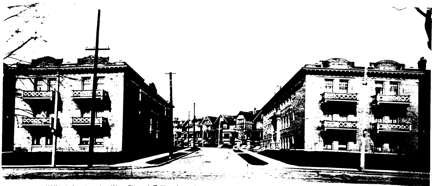
Willard Apartments, King St. and Triller Ave. Henry Simpson, Architect. Holtby Bros., Mason Contractors.
