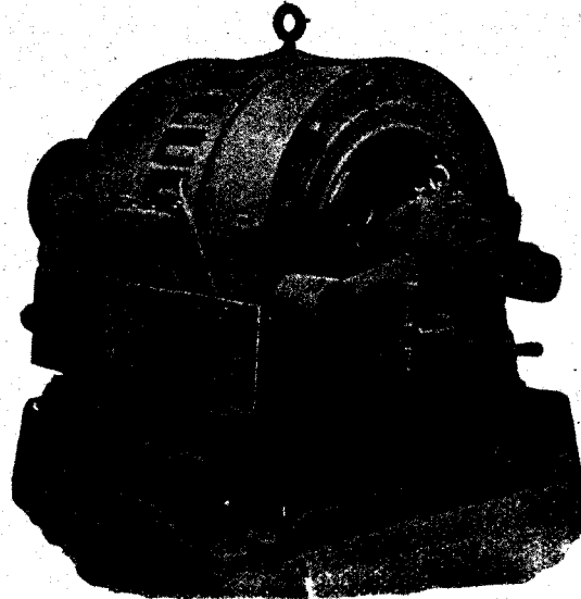
S.K.C. 50 Kilowatt Two-Phase Generator
